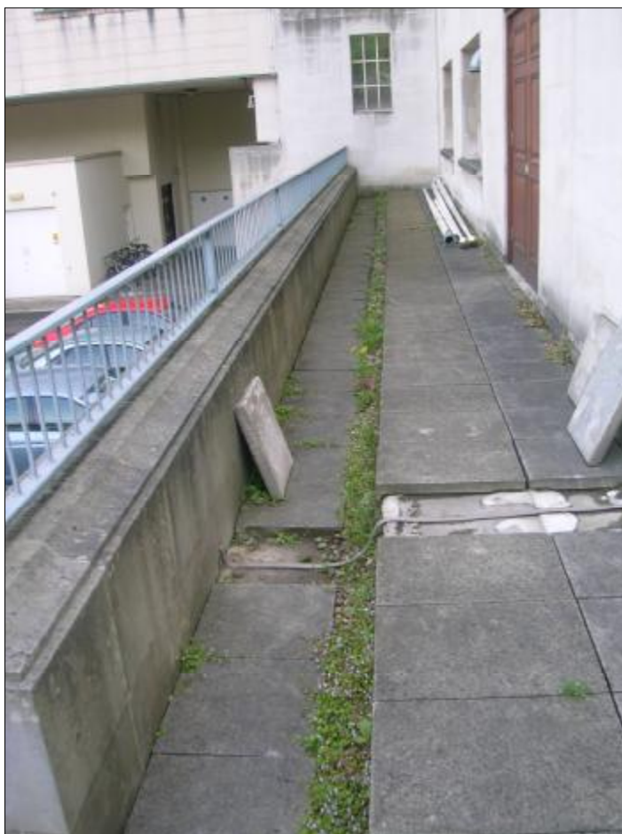
Figure 8. Ephemeral vegetation on French drain above lower car park.
