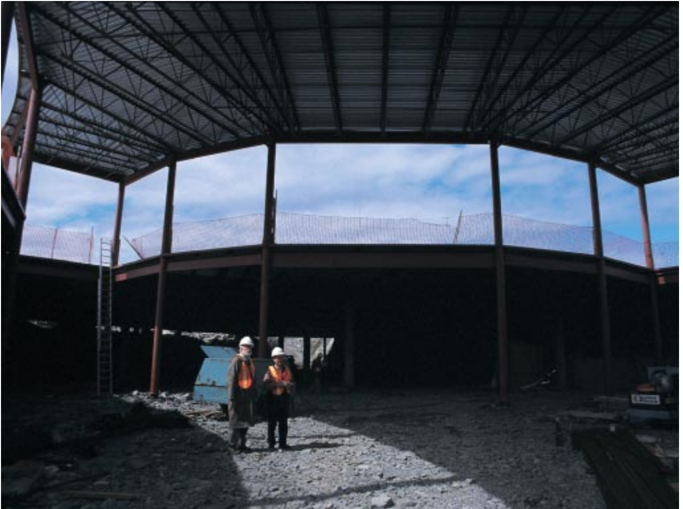
Geocentre under construction, June 2001
