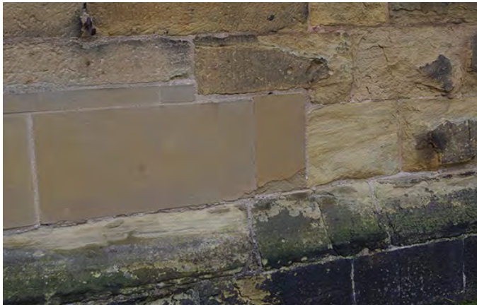
Fig. 4. (top) Gateway to Wynnstay Hall. Fig. 5. (bottom) York Stone replacements, St Mary's Church, Wynnstay.
