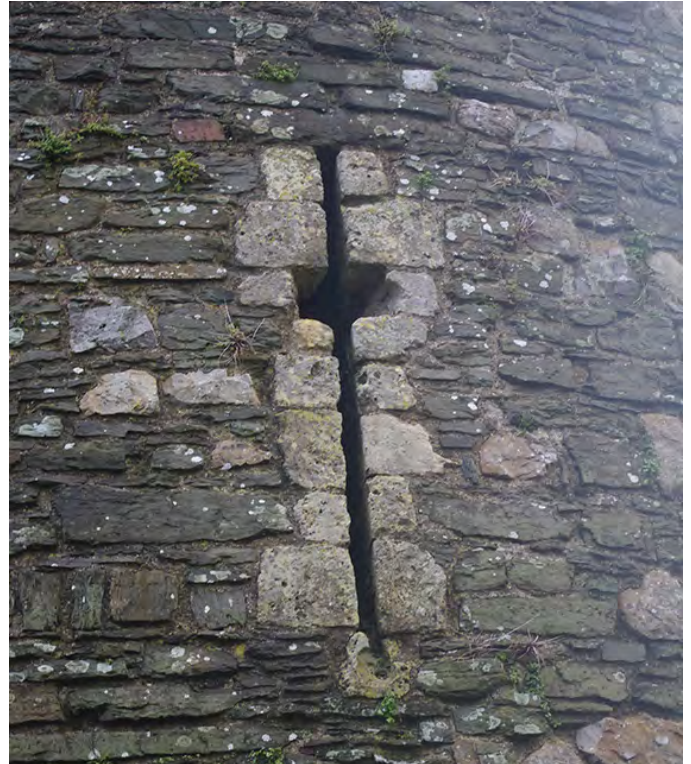
Fig.1 Arrow loops dressed with Sutton Stone, Kidwelly Castle
