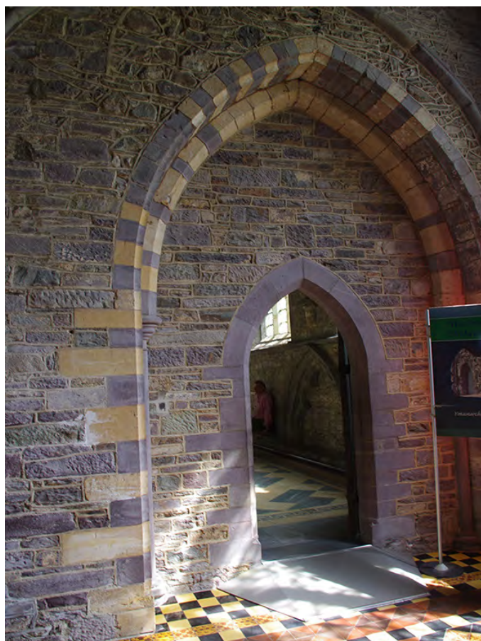
Fig. 4. Caerbwdy Stone and limestone used create a polychromatic effect inside the Cathedral.
