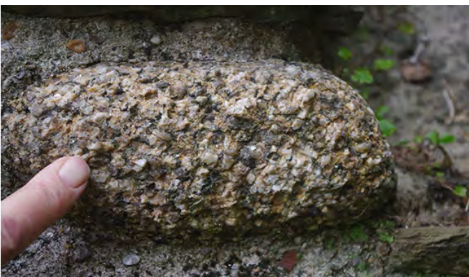
Fig. 2. (top) Badly weathered Quarella Stone in the gatehouse, Kidwelly Castle. Fig. 3. (bottom) Granite boulder in the town wall, Kidwelly.
