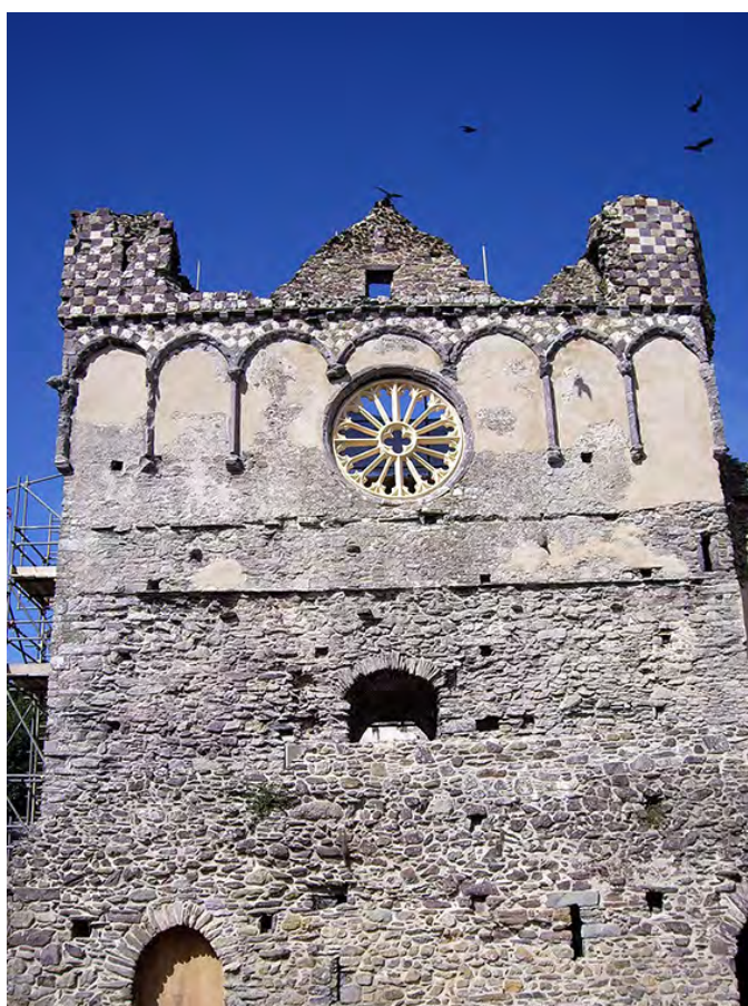
Fig. 5. Different colour tuffs in the Bishop's Palace walling. Fig. 6. The Great Hall east gable of the Bishops Palace.
