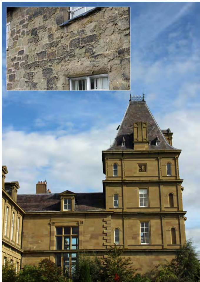
Fig. 3. Good quality Coed yr Allt Sandstone at Wynnstay Hall. (Inset: poor quality stone, Park Street, Ruabon).
