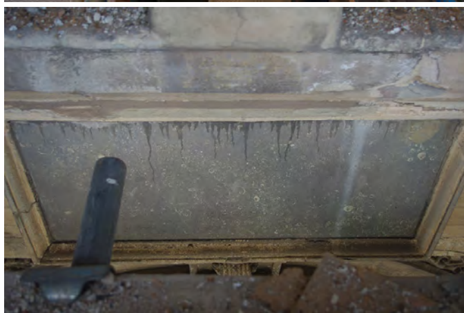
Fig. 1 (top). Members on the scaffolding. Fig. 2. (bottom) Snow-drop Marble, Tredegar House.
