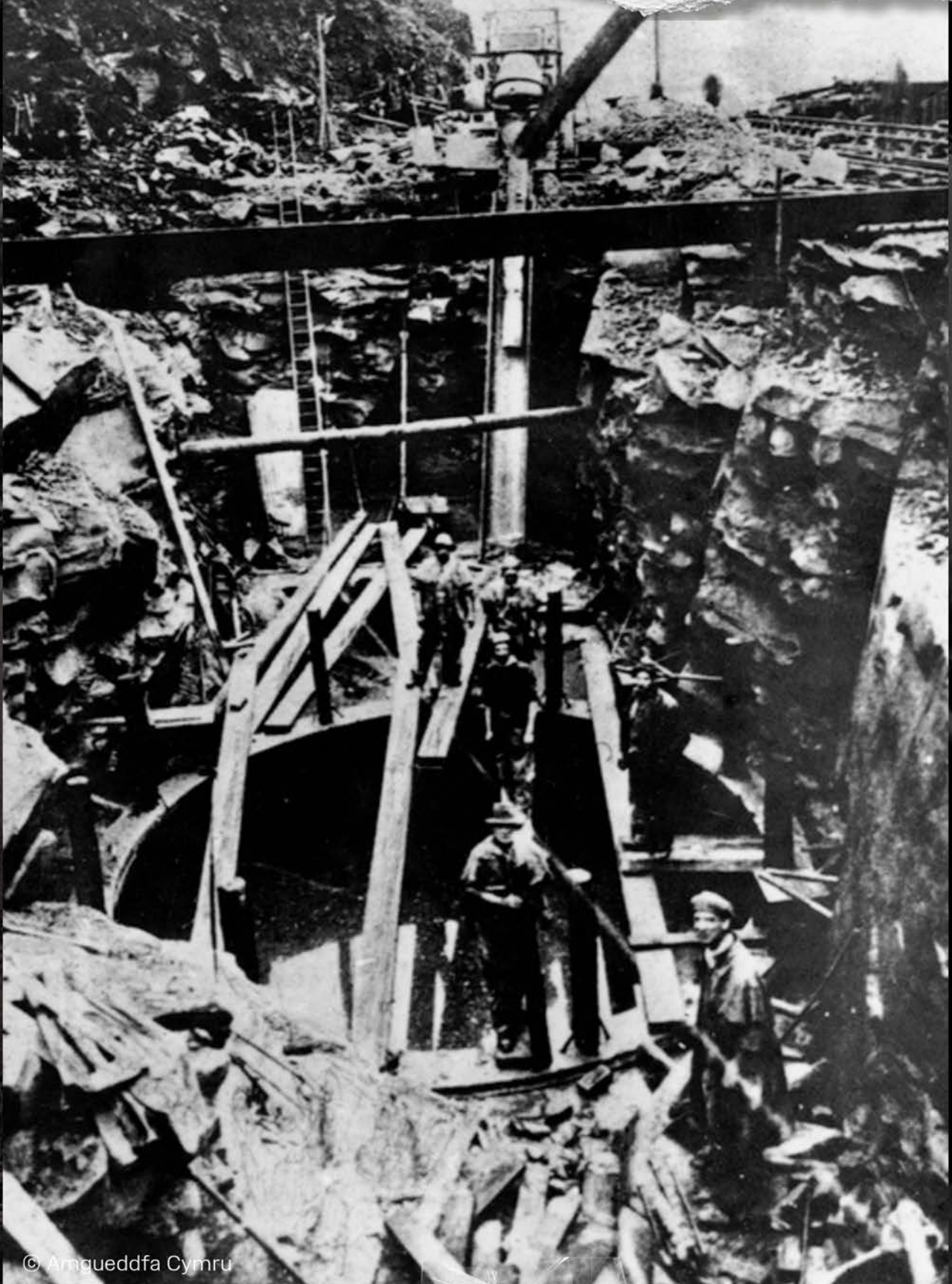
Sinking a shaft, Wyllie Colliery, Pontllanffraith, 1911
