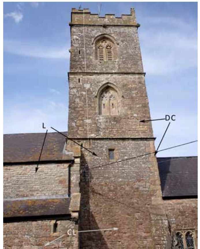
Fig. 7. South face of tower showing reddened Carboniferous Limestone (CL) and Lias Limestone (L) with Dolomitic Conglomerate (DC) quoins. Upper stages of DC with DC quoins.
