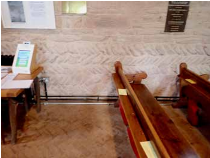
Fig. 3 (above) Herringbone masonry, St. Andrew, Bredwardine. Fig. 4 (top right) St Michael and All Angels, Mocca, fabric of tufa blocks. Fig. 5 (middle right) Detail of yufa blocks show in Fig 4. Fig. 5 (Bottom right) St. Maughan's Formation dressings and tufa block fabric, St. Andrew, Bredwardine. .
