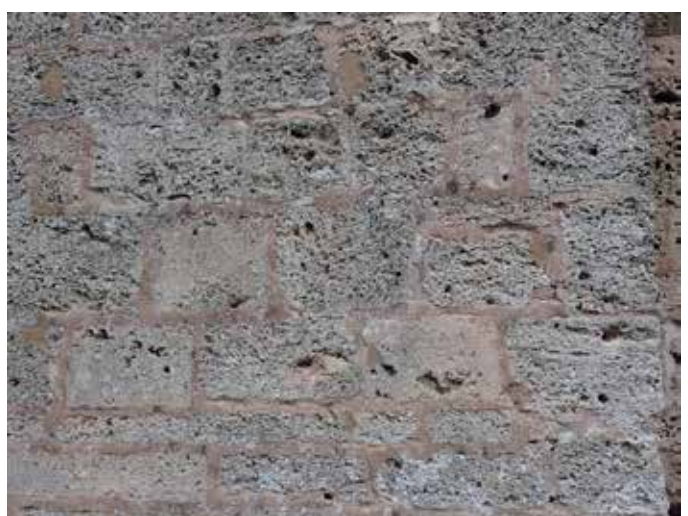
Fig. 3 (above) Herringbone masonry, St. Andrew, Bredwardine. Fig. 4 (top right) St Michael and All Angels, Mocca, fabric of tufa blocks. Fig. 5 (middle right) Detail of yufa blocks show in Fig 4. Fig. 5 (Bottom right) St. Maughan's Formation dressings and tufa block fabric, St. Andrew, Bredwardine. .
