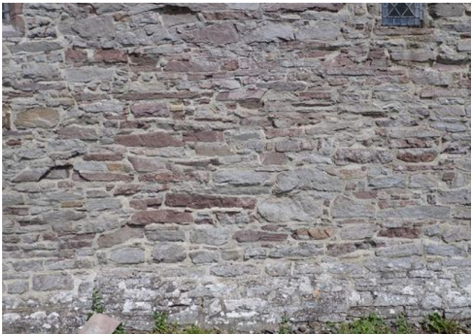
Fig. 1. (top left) St. David's Llanddew, viewed from SE. Fig. 2. (middle left) west wall of vestry showing the west wall of the vestry showing extensive rebuilding. Fig. 3. (bottom left) fabric of chancel wall composed of red and grey rubblework sandstones. Fig. 4. (top right) Rare block of tufa in fabric. Fig. 5. (bottom right) Window, south chancel red and mottled sandstone, replaced during renovation work.
