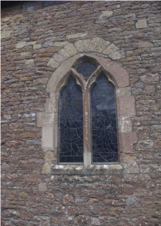
Fig. 21. C14 chancel window of Dolomitic Conglomerate and (later replacement?) Dundry Stone.
