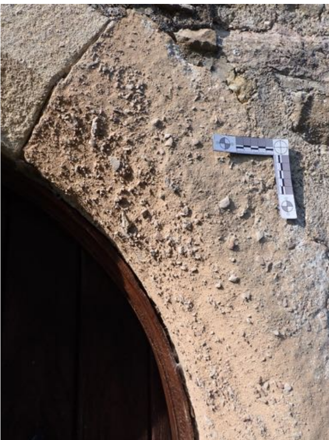
Fig. 3. (top left) South porch of ashlar Dolomitic Conglomerate. Roof of nave behind displaying two shades of grey slate. Fig. 4. (bottom left) Dolomitic Conglomerate from porch ashlar, showing slightly smaller clasts than stone used in earlier medieval dressings. Fig. 5. (top right) West doorway worked in Dundry Stone. Fig. 6. (bottom right) Close up of Dundry Stone in Fig. 5.
