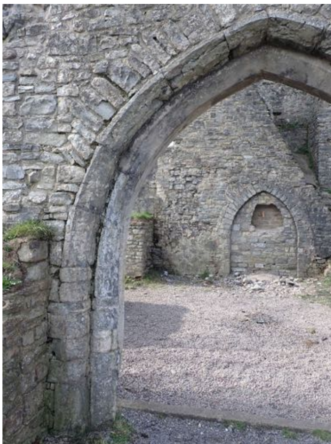
Fig. 1. (top left) General view of St Mary's Caerau, from the NE, showing ruined state. Fig. 2 (left middle) Lias limestone blocks in the base of the west wall of the tower, these are c 15cm x 60cm. Fig. 3.(bottom left) Chancel arch worked from Lias limestone, basal 5-6 blocks, laid with horizontal bedding, the arch with faces bedding. Tower arch of Lias blocks seen in the background. Fig. 4. (top right) southeast corner of nave showing limestone quoins inserted by Pritchard. Long Lias blocks on the east wall of the porch seen in background. Fig 5 (middle right) C19 Bath Stone corbel from the west side of the porch roof.
