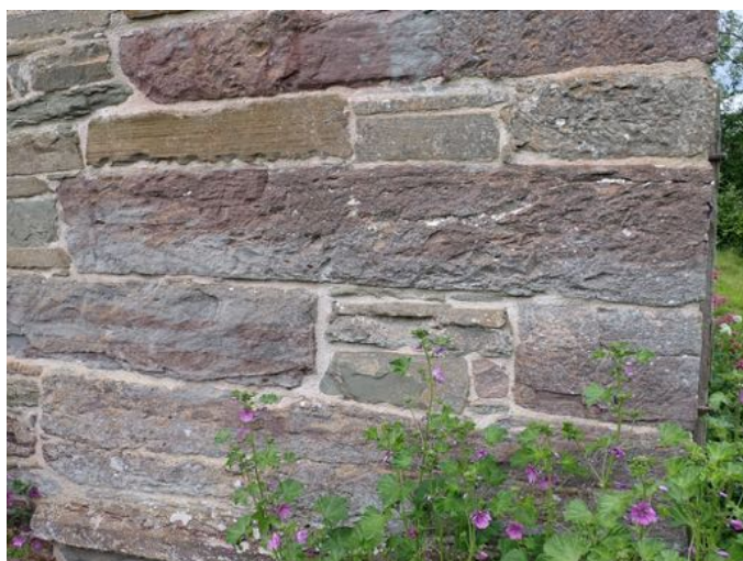
Fig. 10 (top) St. Eigon's church, Llanigon. Fig. 11. (bottom) large slabs of grey/maroon sandstone, south chancel wall.
