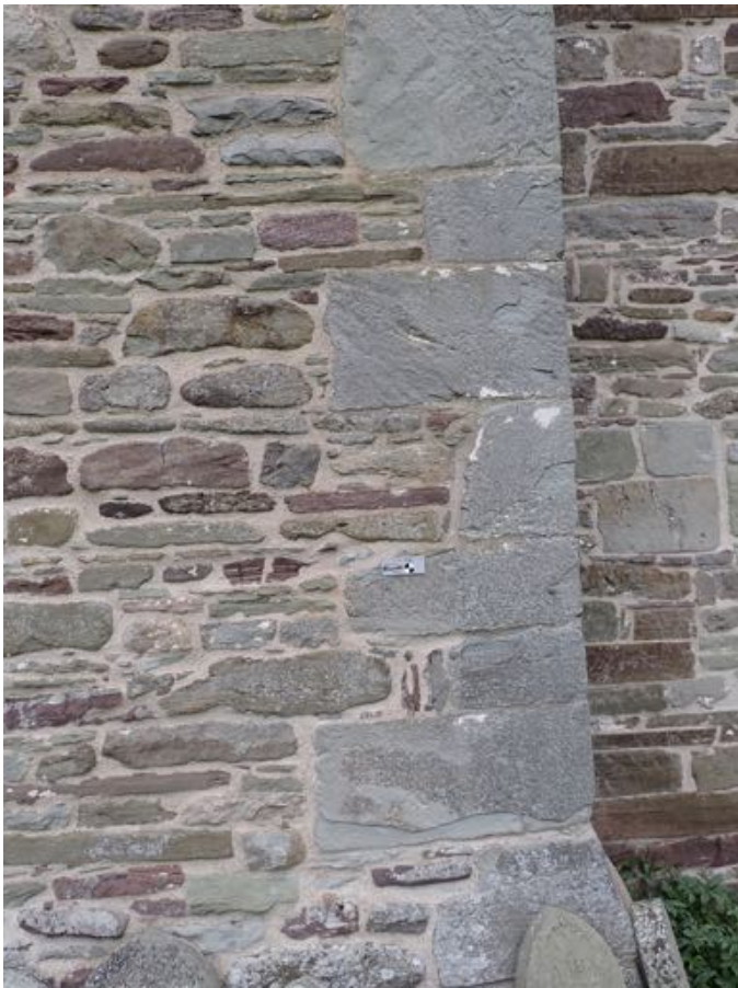
Fig. 14. Grey homogenous sandstone quoins, SE nave, inserted during C19 restoration work.
