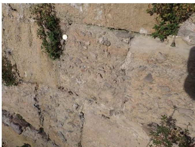
Fig. 24. Ashlar blocks of Sudbrook Stone, in main Gatehouse. Fig. 25. Detail of blocks, showing some to be conglomeratic with coarse angular fragments of limestone. Fig. 26. Block in Gatehouse showing rounded and angular clasts. Fig. 27. Small exposure of Dolomitic Conglomerate, to the west of the Gatehouse, containing angular and rounded clasts
