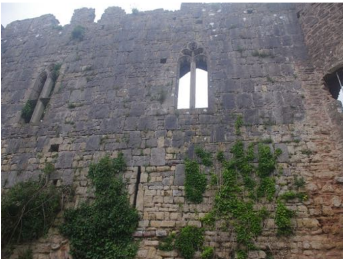
Fig. 28. (top left) Banded yellow and red Sudbrook Stone in arch on S curtain wall. Fig. 29. (top right) Curtain wall by SE tower, showing base composed of Sudbrook Stone (yellow) and upper courses in Carboniferous Limestone (grey). Fig. 30. (bottom left) Coursed blockwork of Sudbrook Stone (SW tower), colour variation a product of battered structure of wall catching greater moisture. Scale provided by our new Treasurer, Heather Jackson. Fig. 31. (bottom right) Close up of Sudbrook Stone showing mottling produced by lense of finer red sand.
