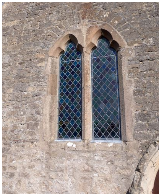
Fig.2. Dolomitic Conglomerate window in west wall.
