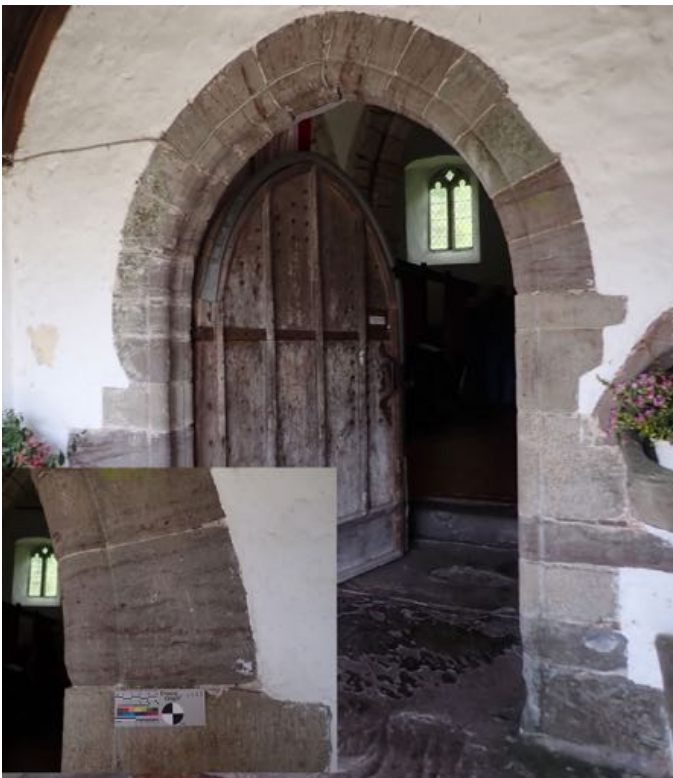
Fig. 6. (top left) St Matthew's church, Llandefalle, viewed from the south. Fig. 7. (bottom left) south doorway, of streaky maroon sandstones, with inset detail showing cross bedding. Fig. 8. (top right) C13 font of red banded sandstones similar to that seen in the south doorway. Fig. 9. (bottom right) faux slate monument with inset showing sandstone composition.
