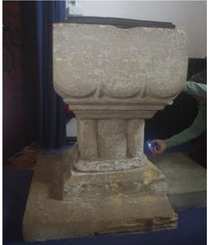
Fig. 7. (top left) south doorway of Dolomitic Conglomerate with some replacement by Bath Stone. Fig. 8. (bottom left) Chancel arch of Sudbrook Stone, stone on middle left shows characteristic yellow/red mottling. Fig 9. (top right) square, C12, font of Sudbrook Stone.
