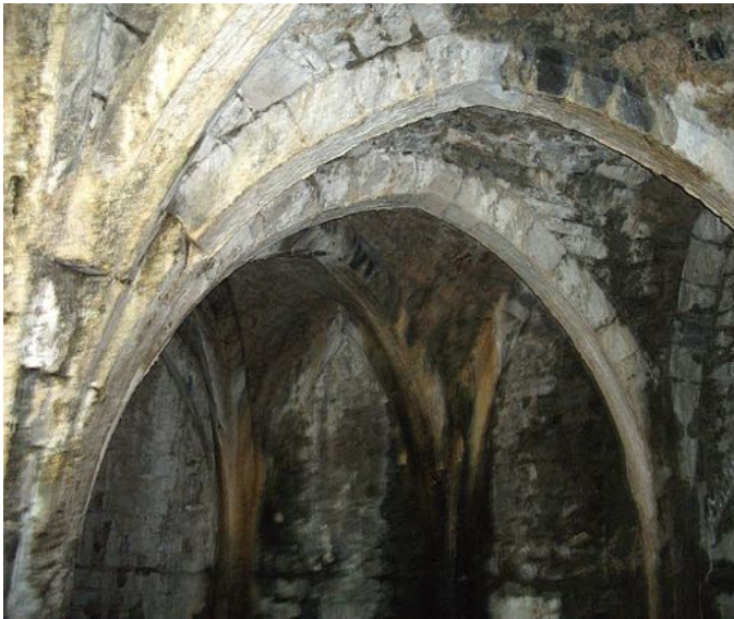
Fig. 5. Ceiling. © Michael Statham
