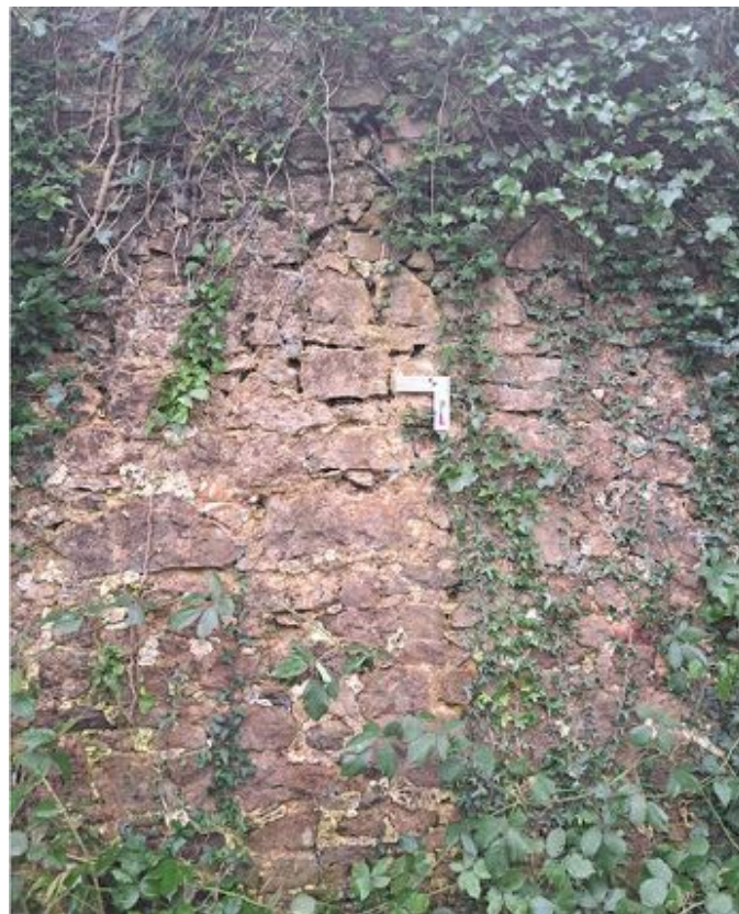
Fig. 8. (bottom left) fabric of Chapel Tal-y-garn composed of Carboniferous Limestone rubble work, with red staining. Fig 9. (bottom right) C13/C14 trefoil east window worked from Sutton Stone.
