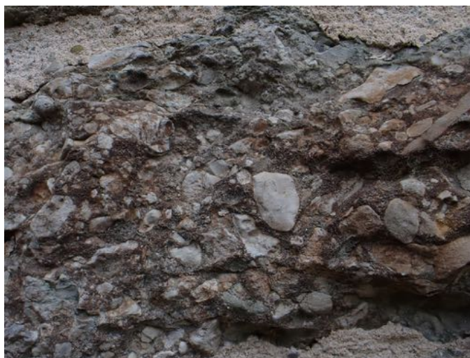
Fig. 12. Calcrete block is rubblework. Fig. 13. Close up of Fig. 12 showing the texture of the carbonate nodules.
