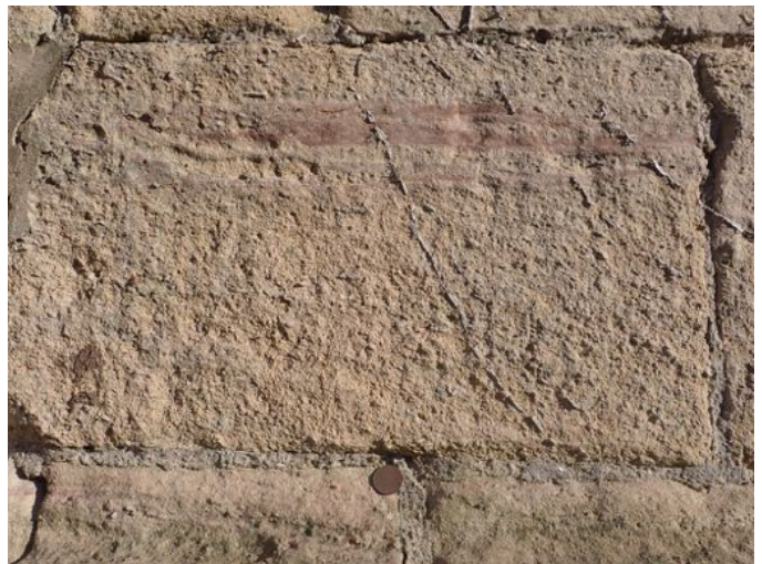
Fig. 28. (top left) Banded yellow and red Sudbrook Stone in arch on S curtain wall. Fig. 29. (top right) Curtain wall by SE tower, showing base composed of Sudbrook Stone (yellow) and upper courses in Carboniferous Limestone (grey). Fig. 30. (bottom left) Coursed blockwork of Sudbrook Stone (SW tower), colour variation a product of battered structure of wall catching greater moisture. Scale provided by our new Treasurer, Heather Jackson. Fig. 31. (bottom right) Close up of Sudbrook Stone showing mottling produced by lense of finer red sand.
