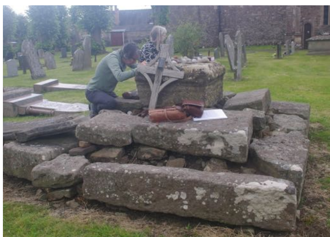
Fig. 11. (top) Medieval socket stone, Dolomitic Conglomerate. Fig. 12. (Bottom) Stepped base (Tintern Stone) and socket stone ?Dundry
