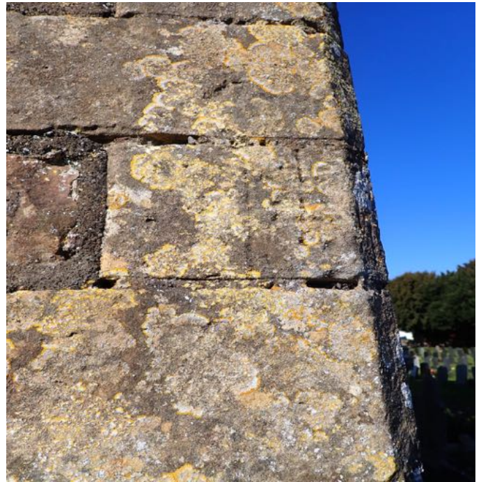
Fig. 19. SE corner of chancel showing Dundry quoins with cross marking.
