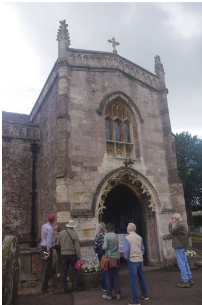
Fig. 13. Porch, St Mary's Magor. Window, outer arch of doorway, and replaced stone below window, Bath Stone. Ashlar; Dolomitic Conglomerate, Dundry Stone, Sudbrook Stone, with minor red 'Tintern Sandstone'.
