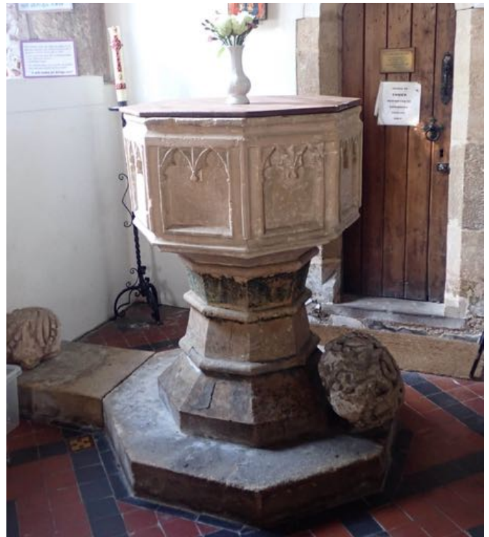
Fig. 23. Dundry Stone font with C19 Bath Stone repairs.
