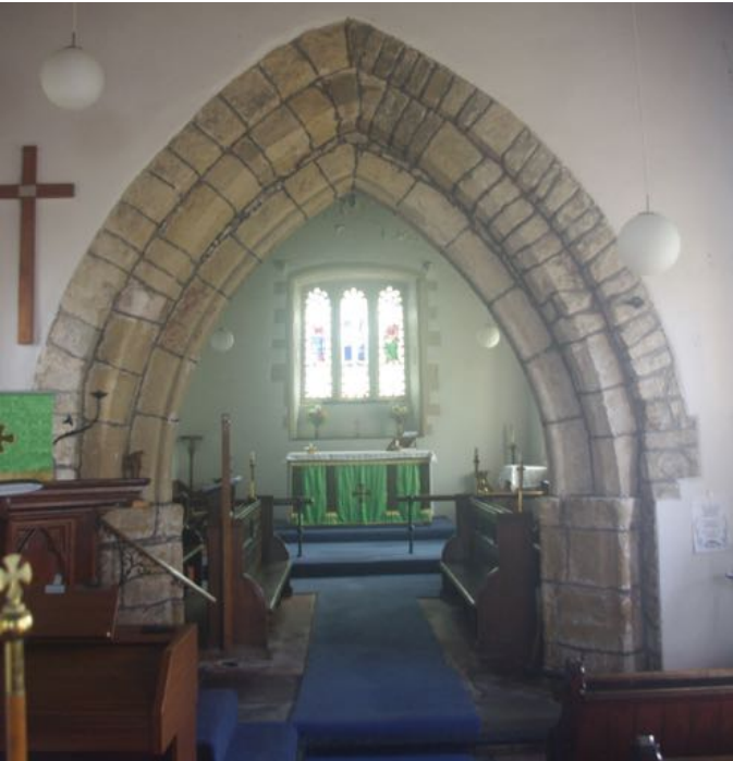
Fig. 7. (top left) south doorway of Dolomitic Conglomerate with some replacement by Bath Stone. Fig. 8. (bottom left) Chancel arch of Sudbrook Stone, stone on middle left shows characteristic yellow/red mottling. Fig 9. (top right) square, C12, font of Sudbrook Stone.
