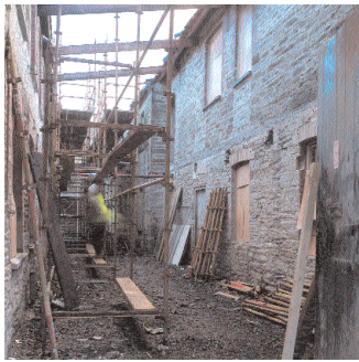
Above: the roof of the yard at the Museum of the Welsh Woollen Industry is removed. It will be replaced with a modern 'glass lid'
